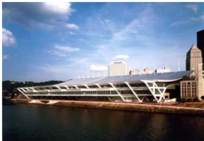
Burt Hill provided engineering and sustainable design services for the David L. Lawrence Convention Center – the largest LEED Gold certified building in the U.S.
